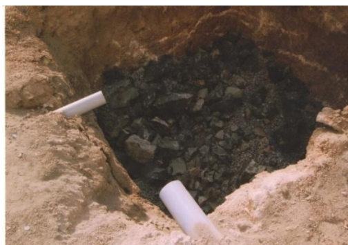
Fig - Recharge Pit of 5x5x7 feet near borewell
