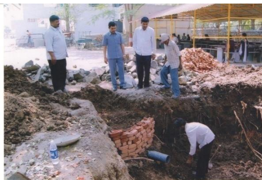
Fig - Recharge Filter bed (15x15x10) near dugwell
