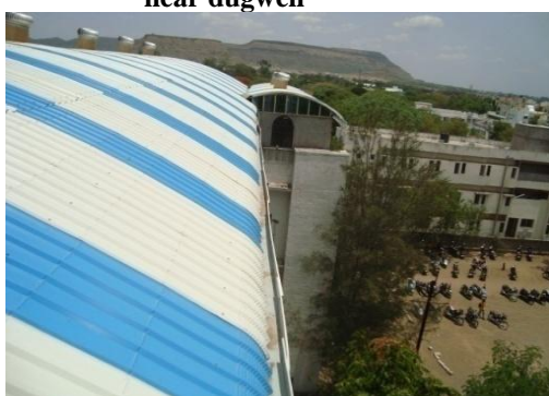
Fig - Roof Water Harvesting in College building
