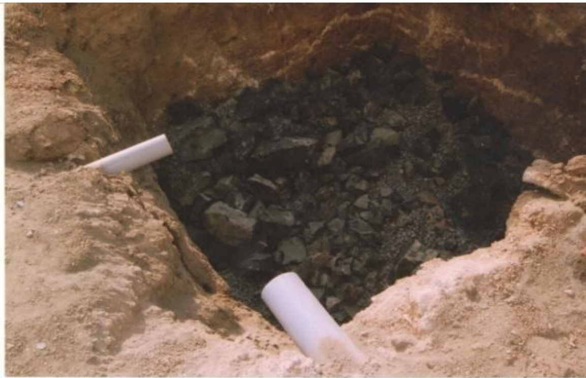
Fig 2:- Recharge Pit of 5x5x7feet near Bore Well
