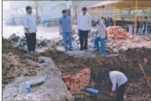
Recharge Filter bed (15 x 15 x 10) near dugwell
