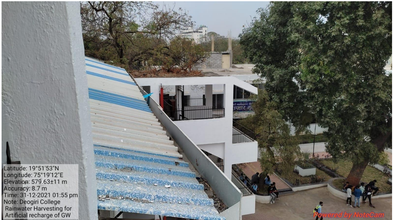
Fig 7:- Roof water harvesting of College building for artificial recharge of bore well / dug well
