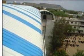
Roof Water Harvesting of College Building
