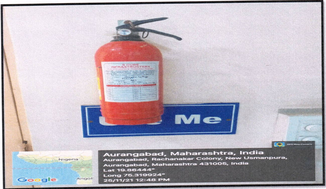
At Science Building Second Floor
