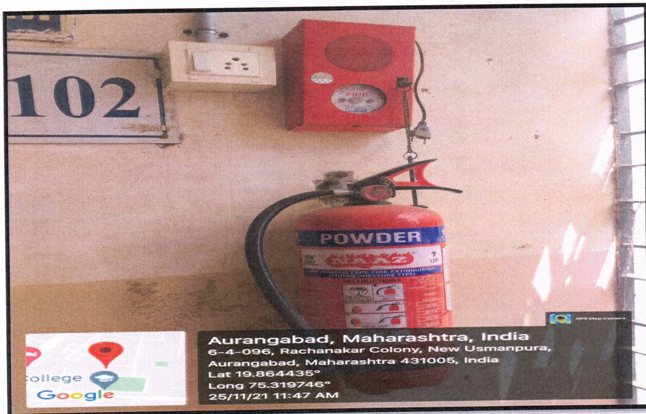
At Commerce Building Second Floor
