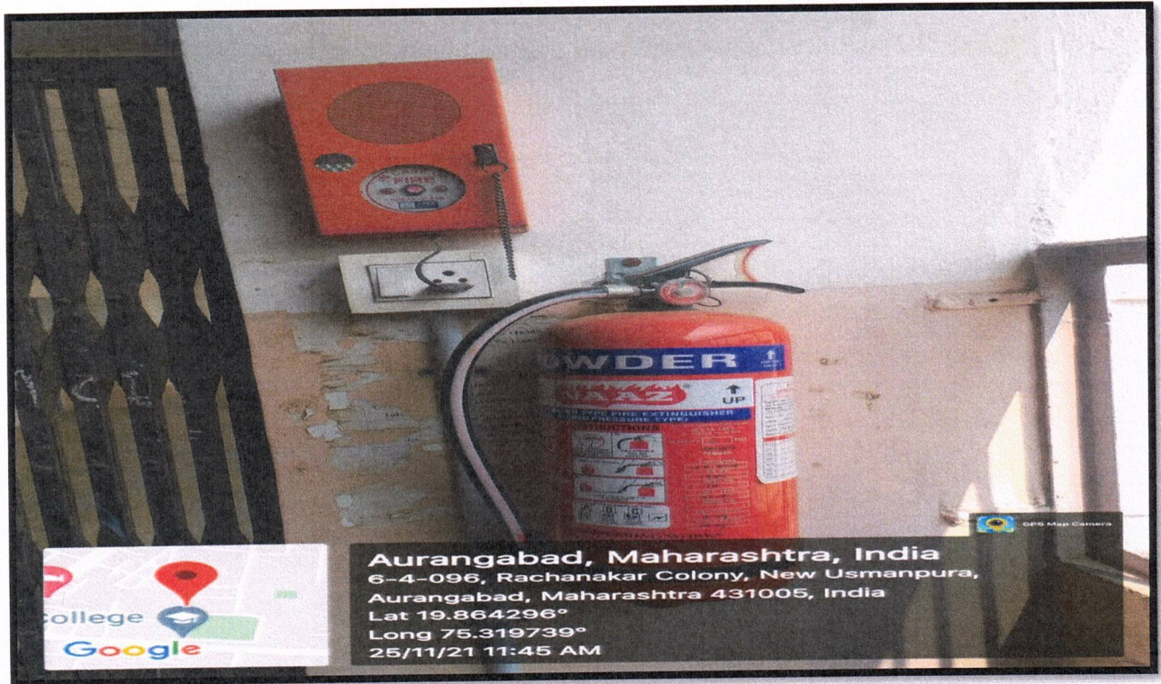
At Commerce Building First Floor
