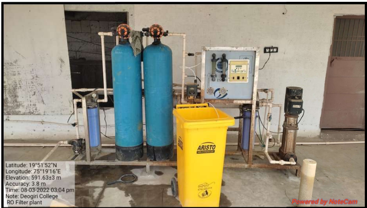
Fig 6:- Ro filter plant
