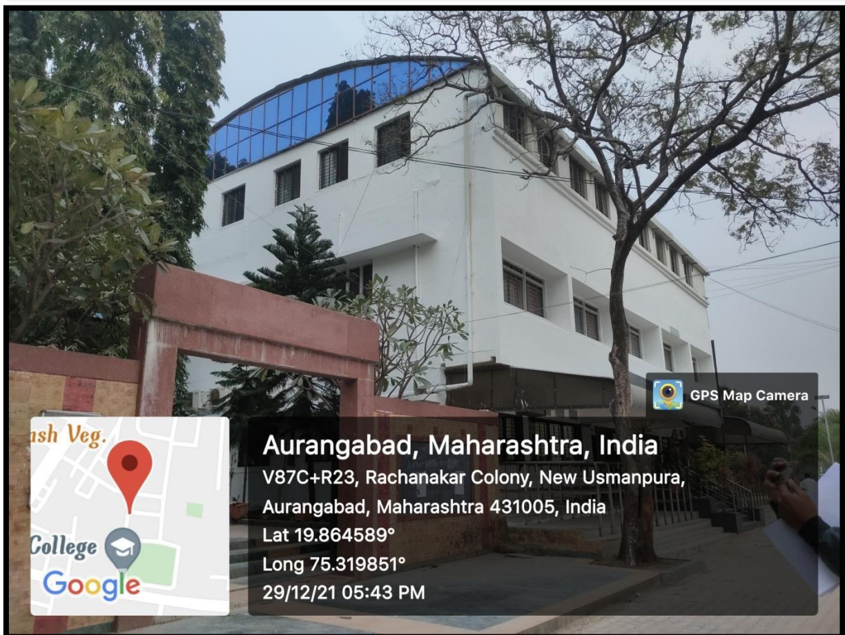
Fig. 11 and 12 - Rainwater Conduit Pipelines on College building
