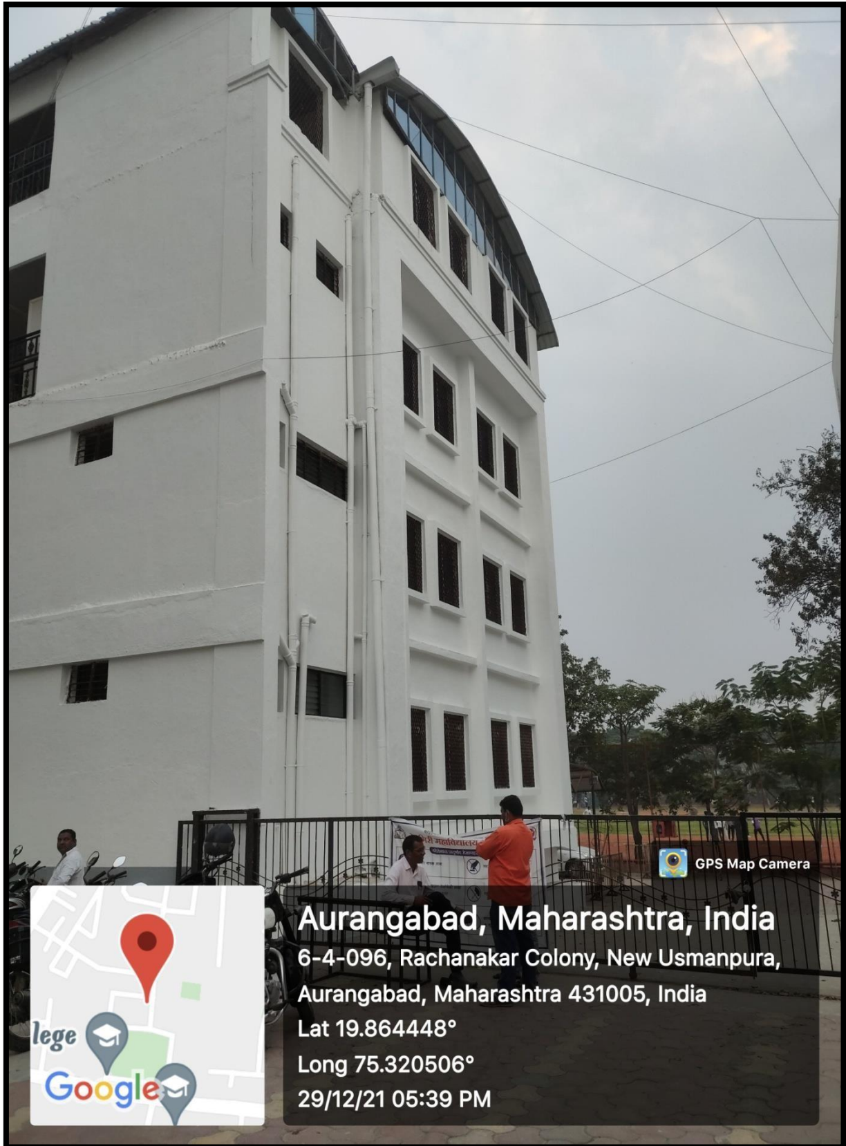
Fig. 08 - Rainwater Conduit Pipelines on College building
