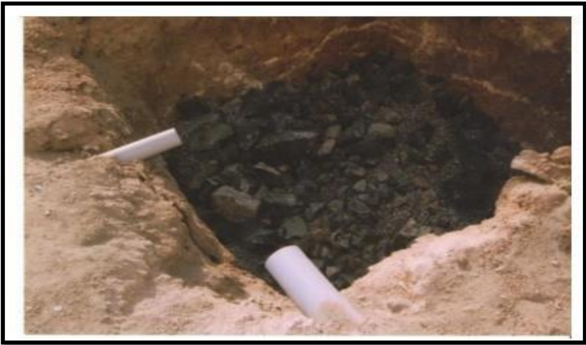
Fig 03 - Recharge Pit of 5x5x7 feet near bore well
