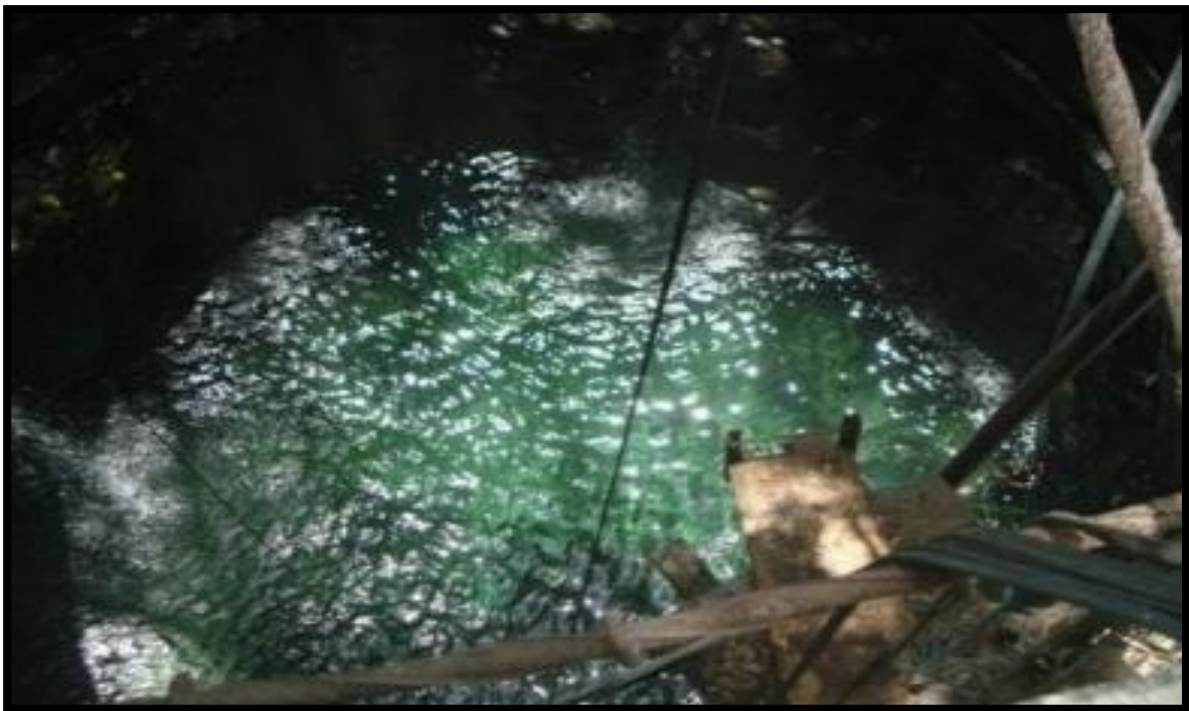
Fig 03 - Recharge Pit of 5x5x7 feet near bore well
