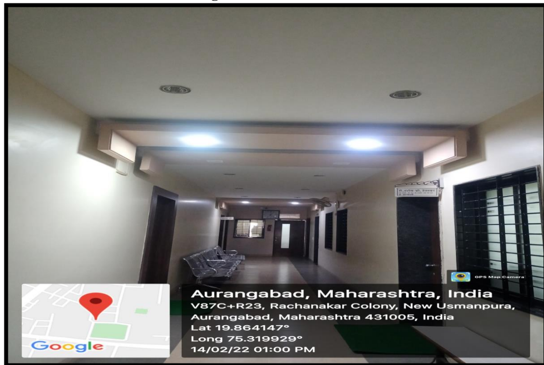
LED lights used in office corridor
