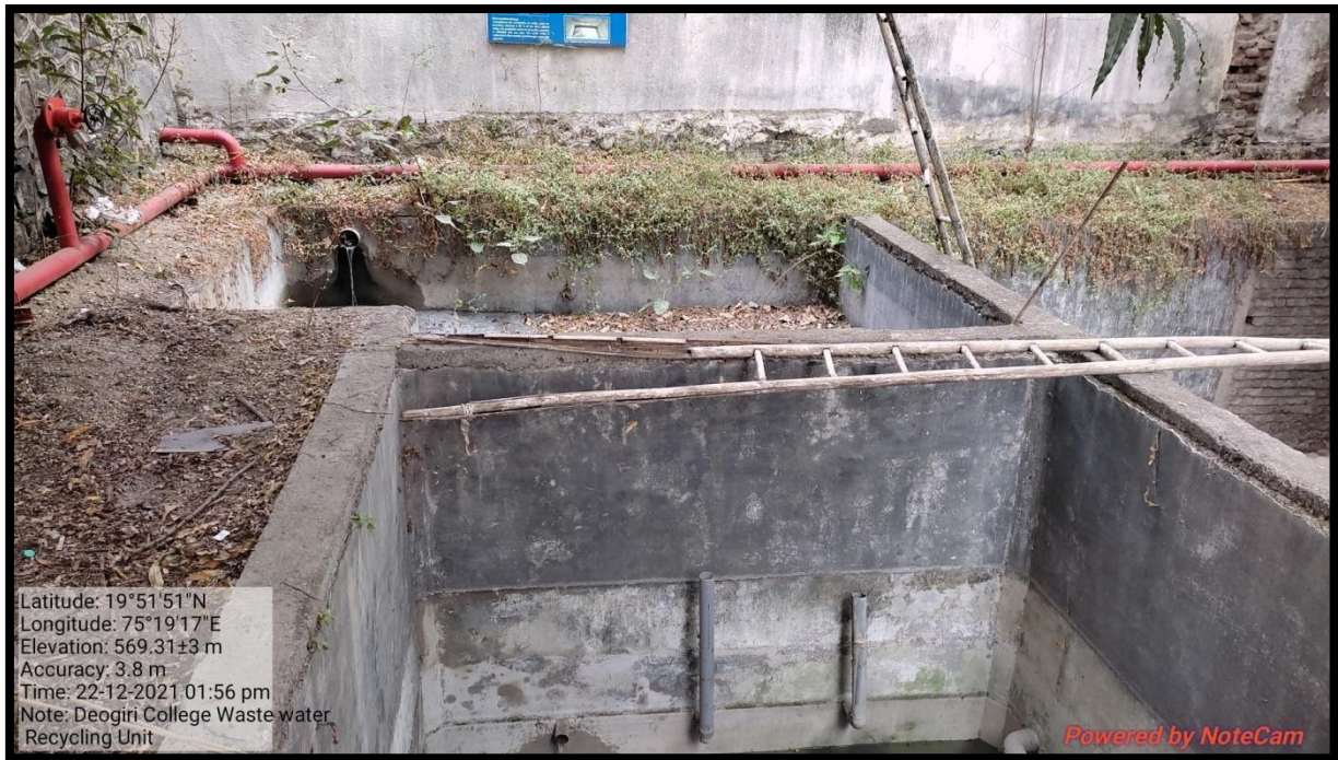
Fig 02:- Water recycling unit.
