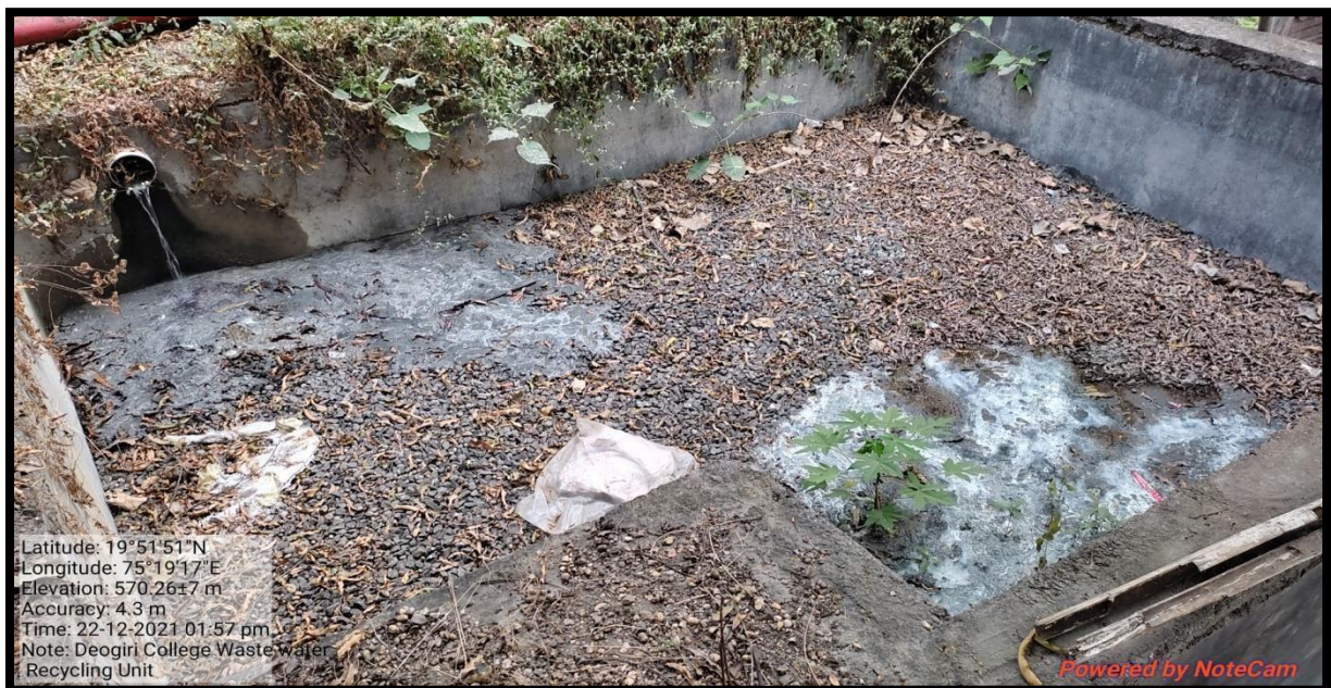
Fig 03:- Solid waste Collector pit of water recycling unit.
