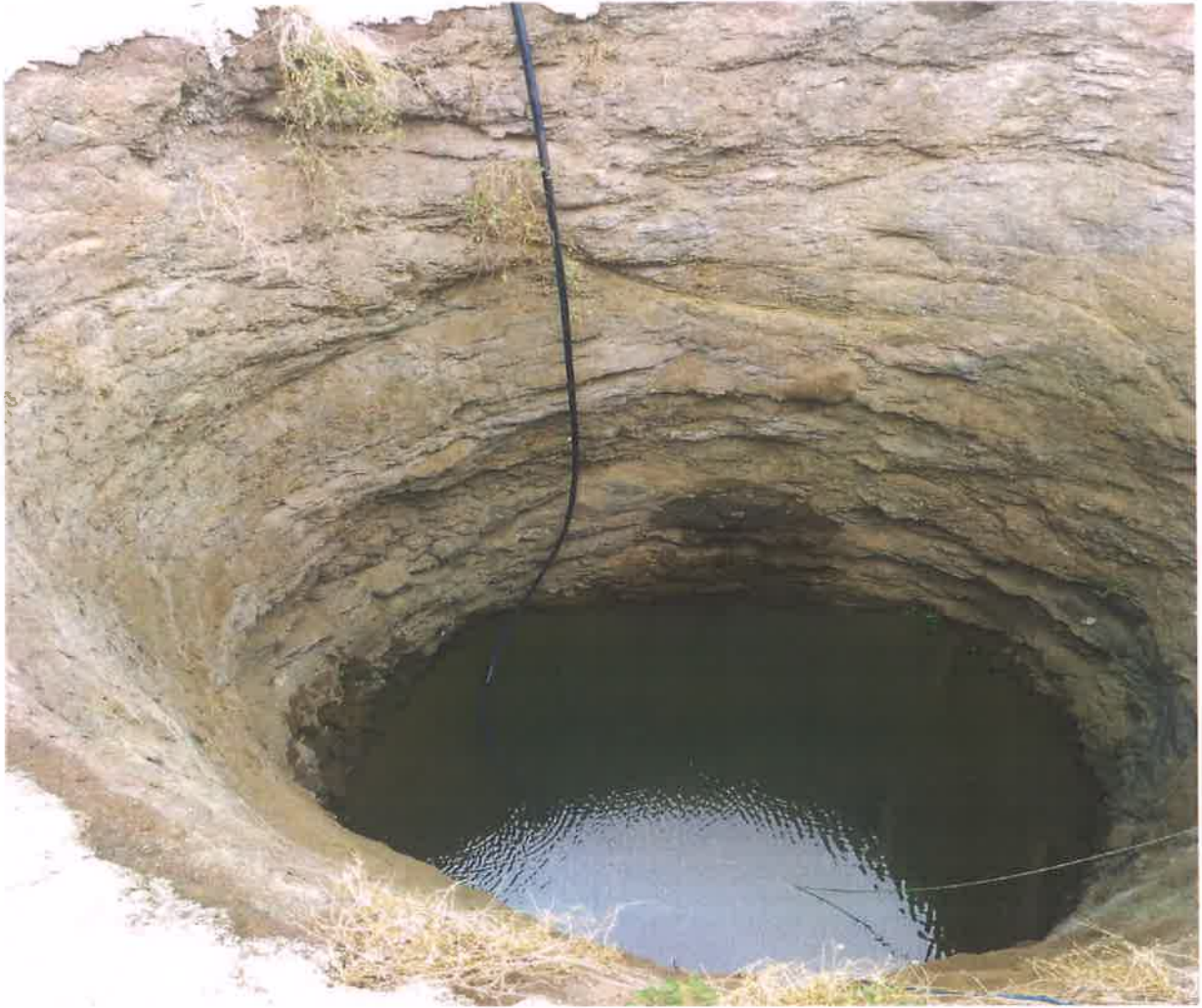
Photographs showing increase in water level at Kinhi village due to watersheds management work.
