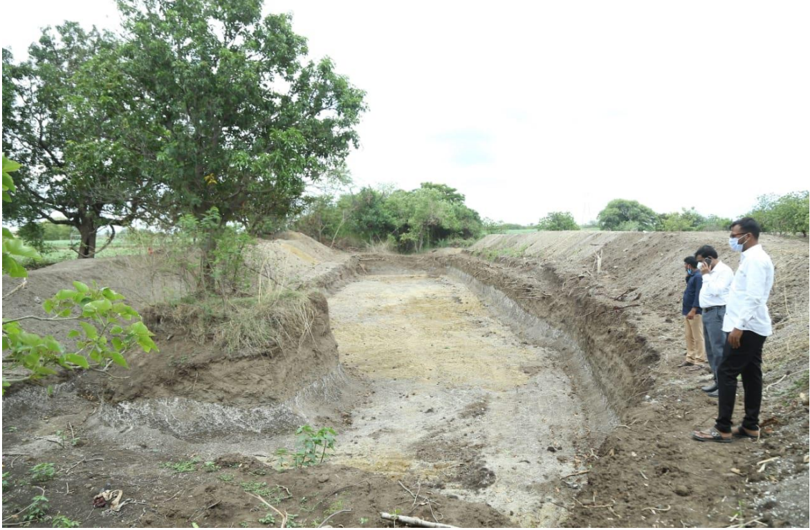
Deeping & Widening of Nala at Pandhri Village
