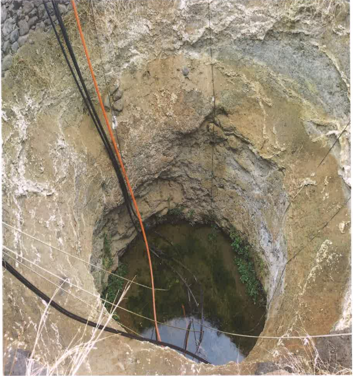
Weathered Compact Basalt Flow with Kanker Deposit
