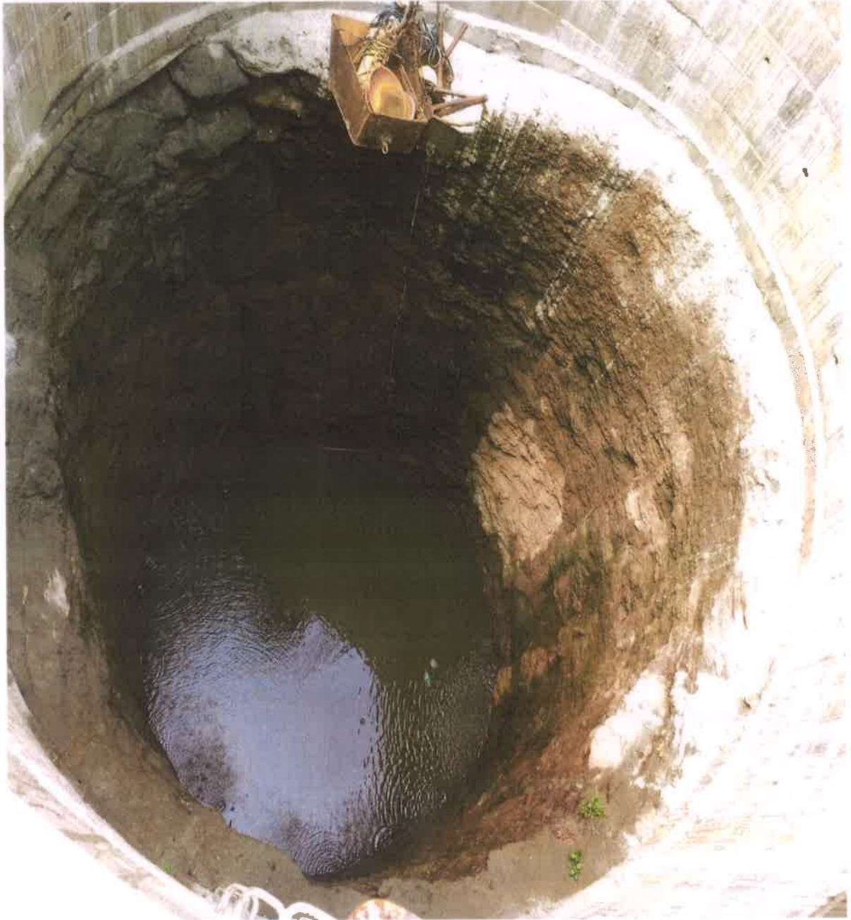
Percolation of water can be seen from the cracks and fractures of the Basalt Flow
