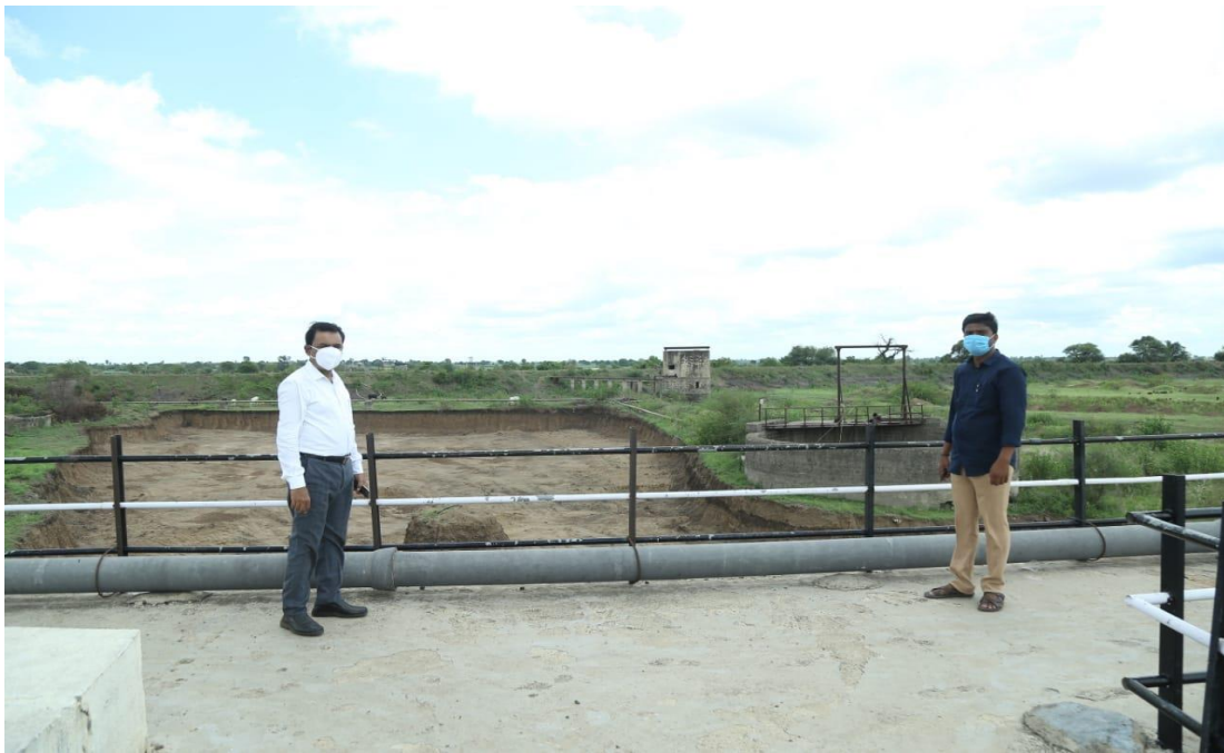
Water Management Work at Rui-Imangaon
