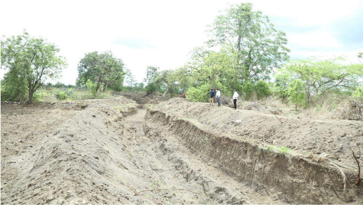
Deeping & Widening of Nala at Pandhri Village
