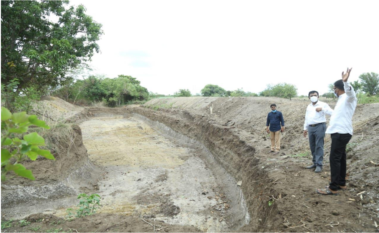
Deeping & Widening of Nala at Pandhri Village
