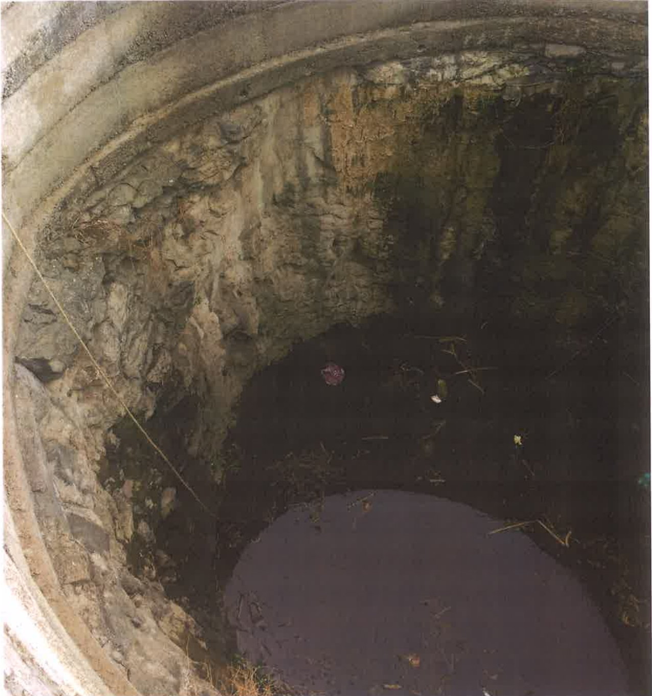
Fractured Compact Basalt can be seen in dug well
