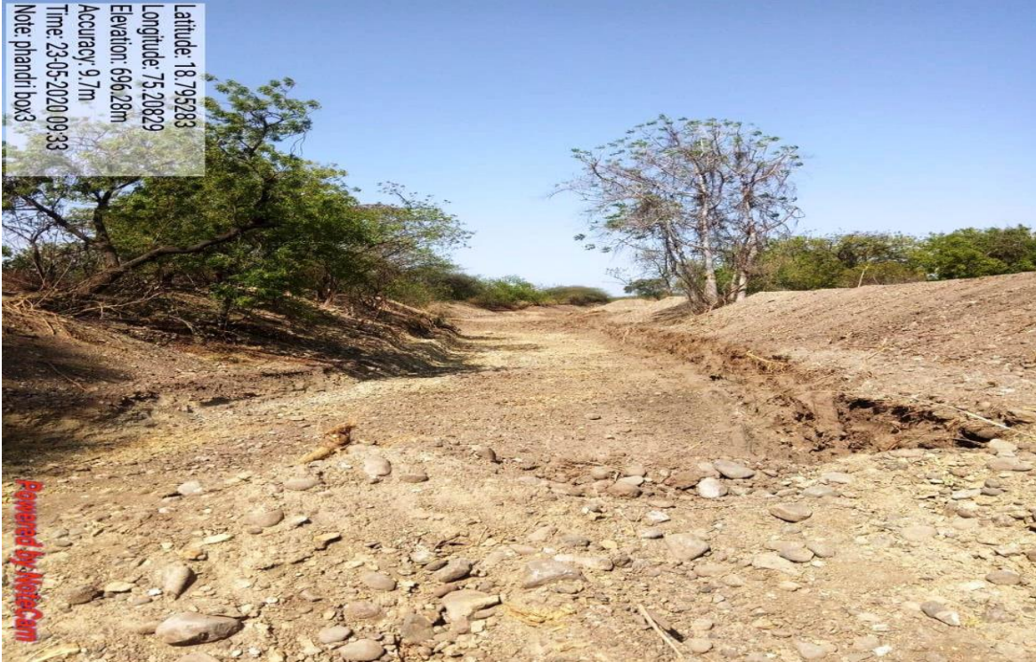
Deeping & Widening of Nala at Pandhri Village
