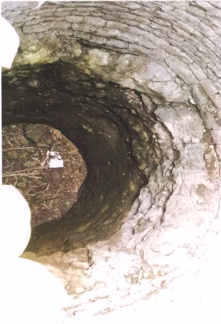
Weathered Compact Basalt Flow can be seen below the stone lining
