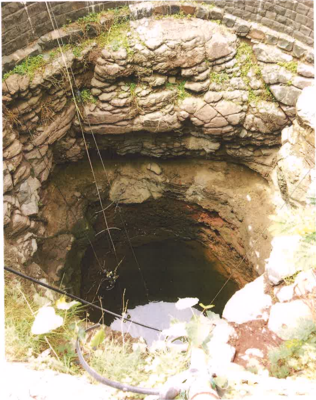
Weathered basalt exposed in dug well below the stone lining
