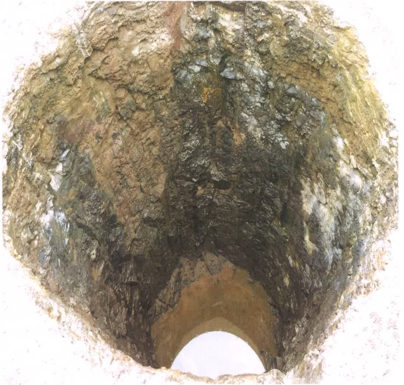
Fractured Compact Basalt in which percolation of water can be seen
