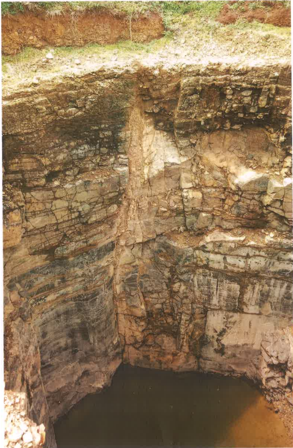
Broadly spaced jointed Compact Basalt Flow can be seen in the outcrop
