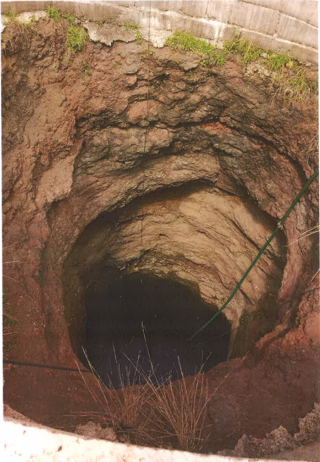
Weathered Compact Basalt is exposed in the dug well
