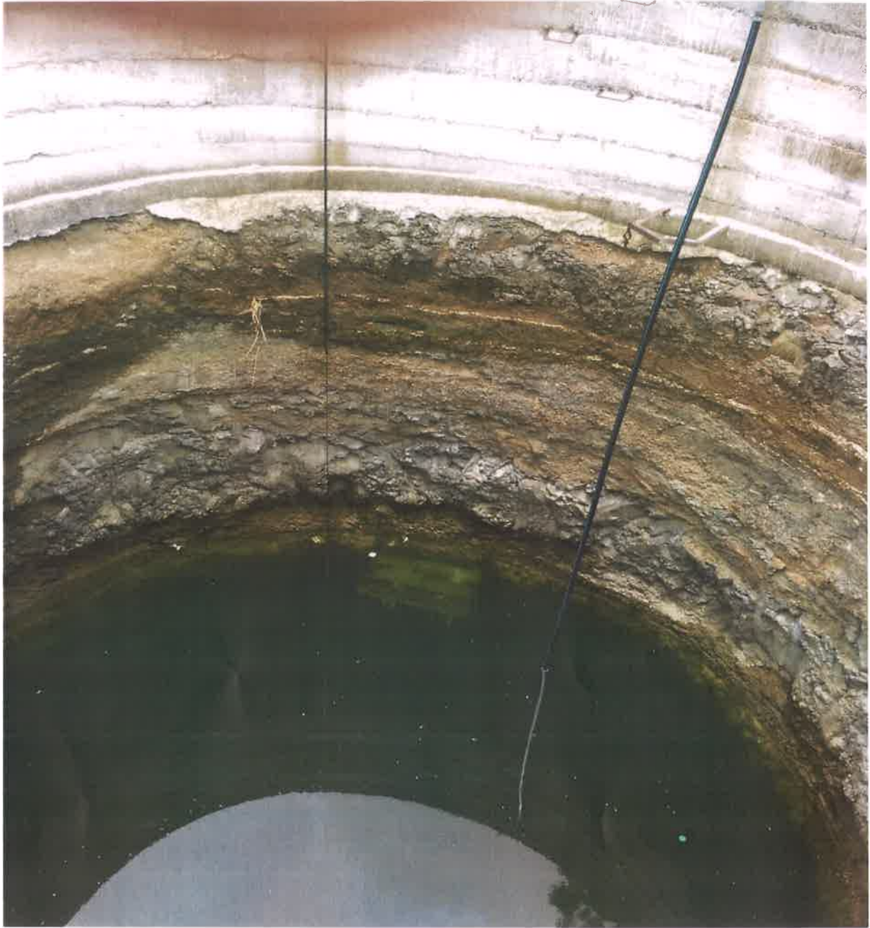
Photographs showing Increase in water level at Devlai.
